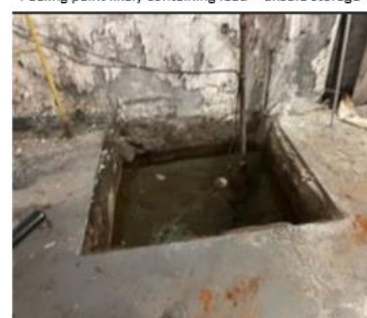
Fall hazard – opened pit in floor
