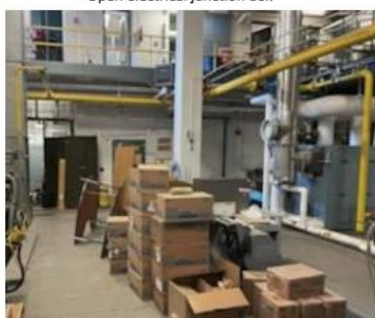
Unsafe storage in mechanical room
