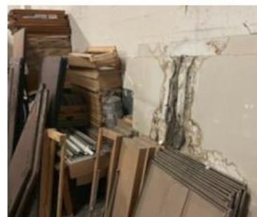
Peeling paint likely containing lead – unsafe storage
