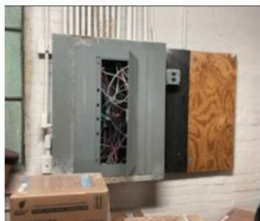
Open electrical junction box
